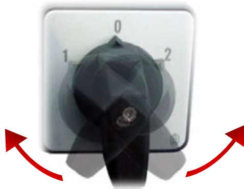
Figure 4. Main Control Switch
